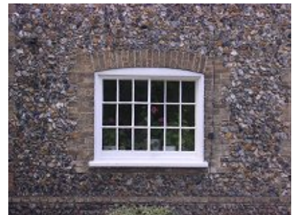
Example of a sliding sash
