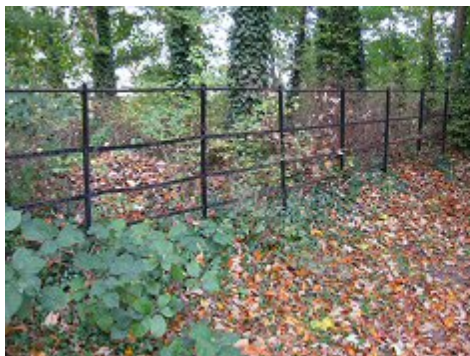
Example of park or estate railings
